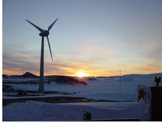
Fig. 7. Alternative power supply options. (left) - Photovoltaic array installed for PLATO, a site testing observatory at Dome A. This nominally 1kW installation uses six panels each rated at 165W, and delivers approximately 200W mean power, integrated over a year (photo - Xu Zhou and Zhenxi Zhu, PLATO deployment team). (right) - One of two 300kW wind turbines at Mawson. (photo – AAD)
