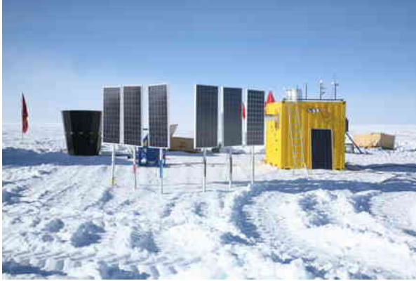
Fig. 7. Alternative power supply options. (left) - Photovoltaic array installed for PLATO, a site testing observatory at Dome A. This nominally 1kW installation uses six panels each rated at 165W, and delivers approximately 200W mean power, integrated over a year (photo - Xu Zhou and Zhenxi Zhu, PLATO deployment team). (right) - One of two 300kW wind turbines at Mawson. (photo – AAD)
